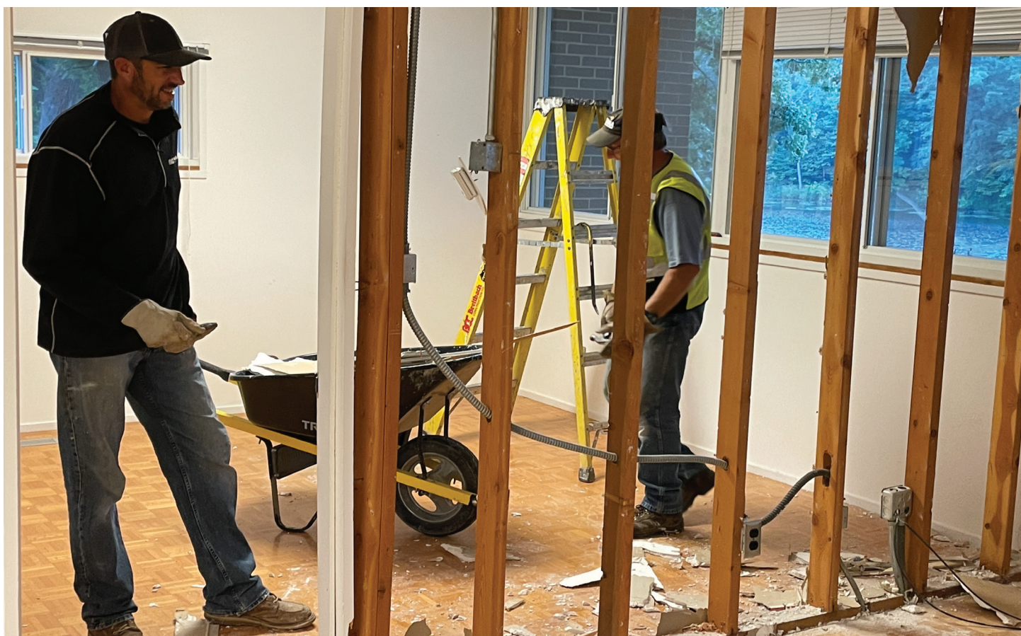
Demolition in the Butler Center is underway!
